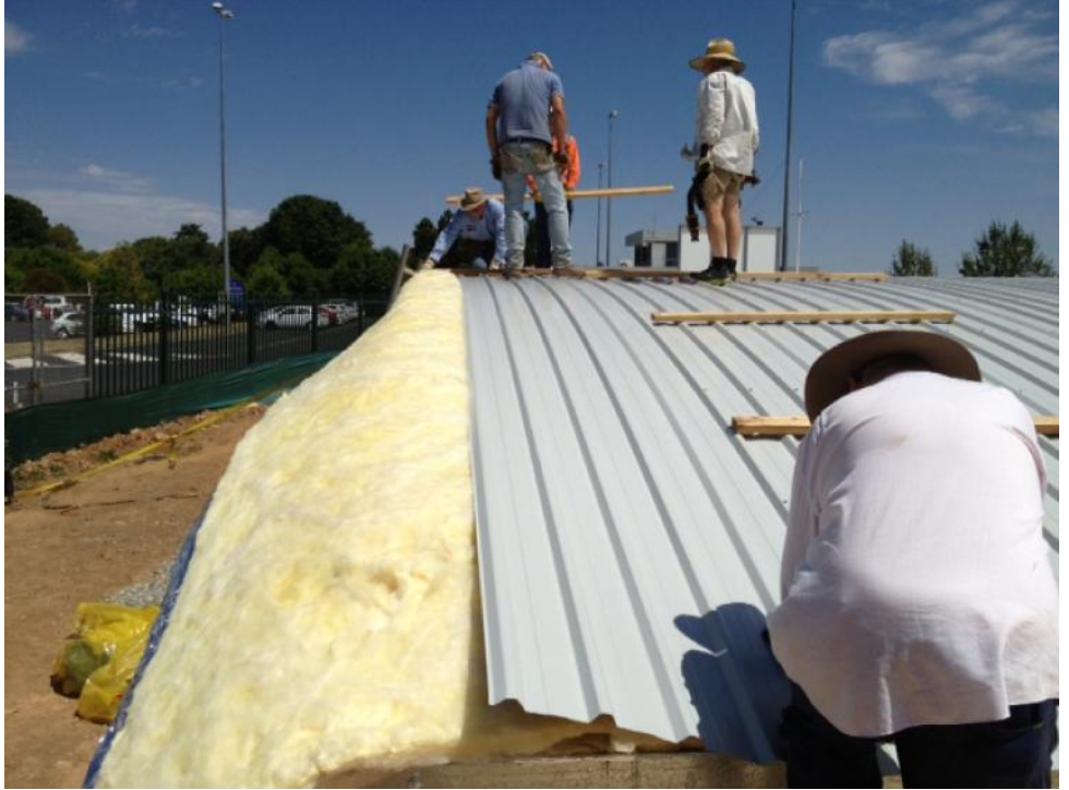
The second-last sheet gets screwed in position
