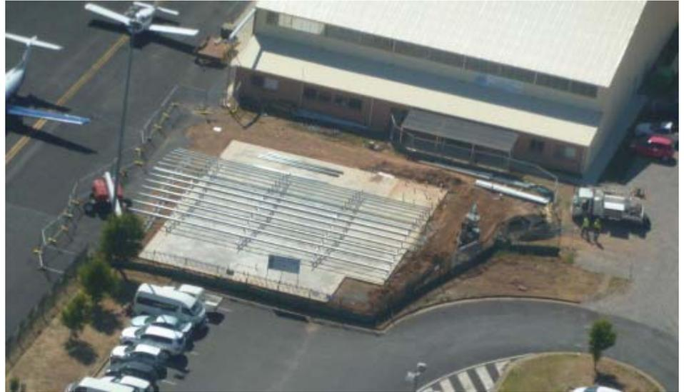
level, which is a much safer and quicker method than erecting the frame first, then sheeting the roof in the air.
