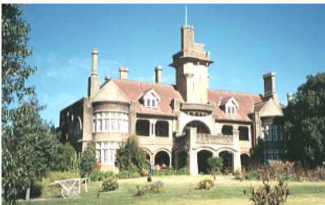
The front view of Iandra Castle showing the irregular tower structure. Should have the flag flying though!
