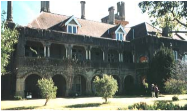
The eastern facade of Iandra Castle
